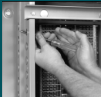
5. Remove knockout plugs from panel.
