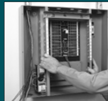
4. Insert interior into tub
