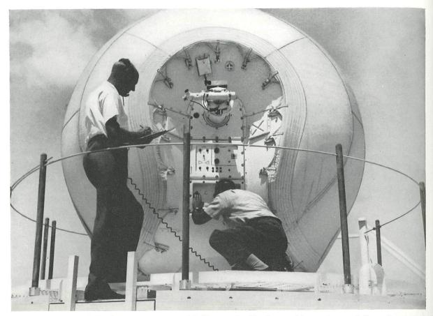
J. C. Crowley and R. J. Tellman check level indicators inside the tracking antenna at Cape Canaveral.
