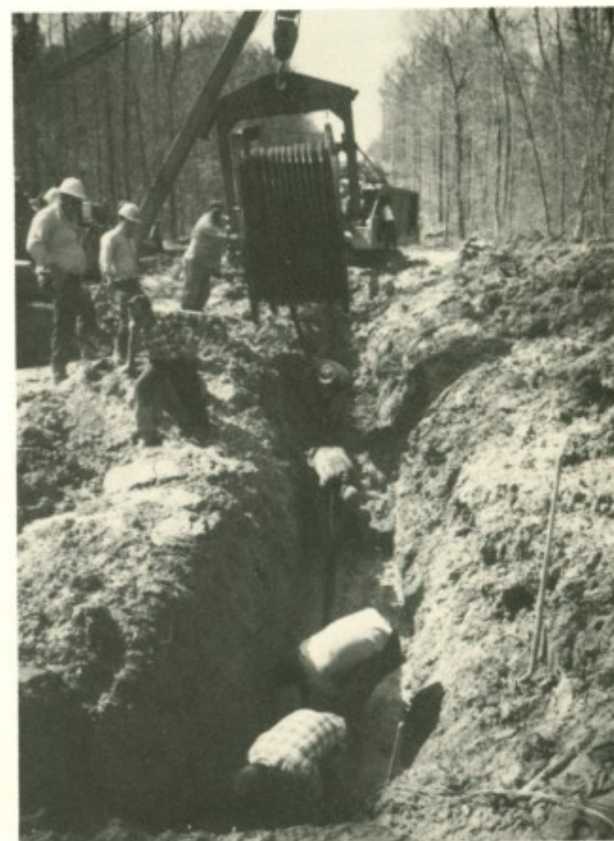
Laying the transcontinental cable through West Virginia on the Monrovia-Williamstown route.
