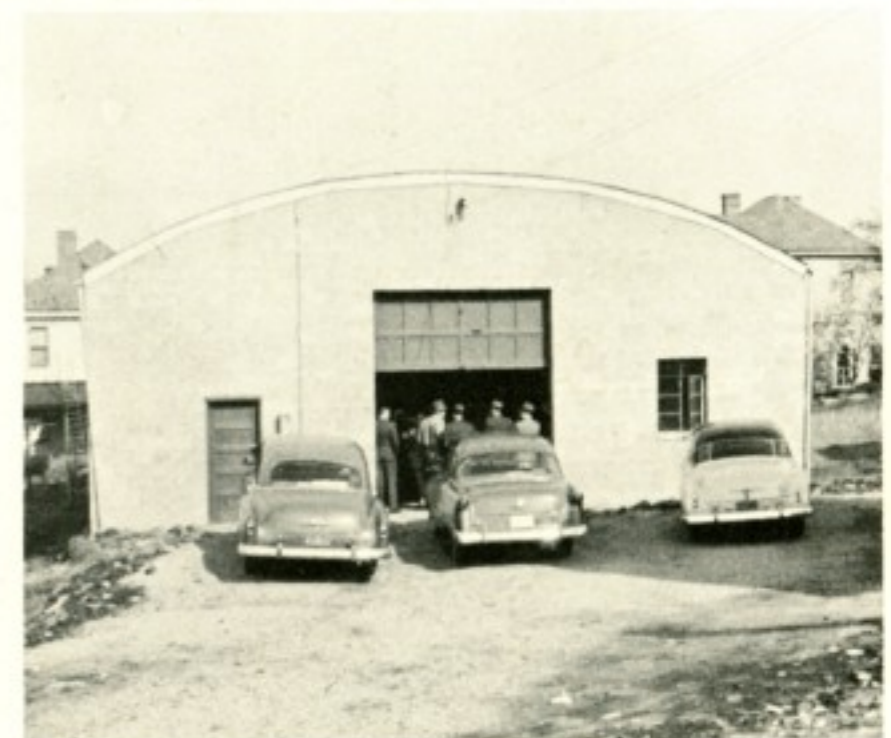
Clarksburg, W. Va. storeroom in 1952
