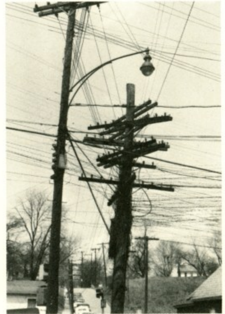
Old Cumberland-Parkersburg open wire line in Bridgeport, W. Va. around 1950.
