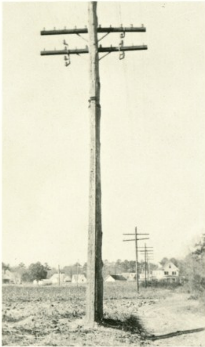
Square pole on the Richmond-Norfolk section of the Norfolk-Washington line installed in 1897-1898.
