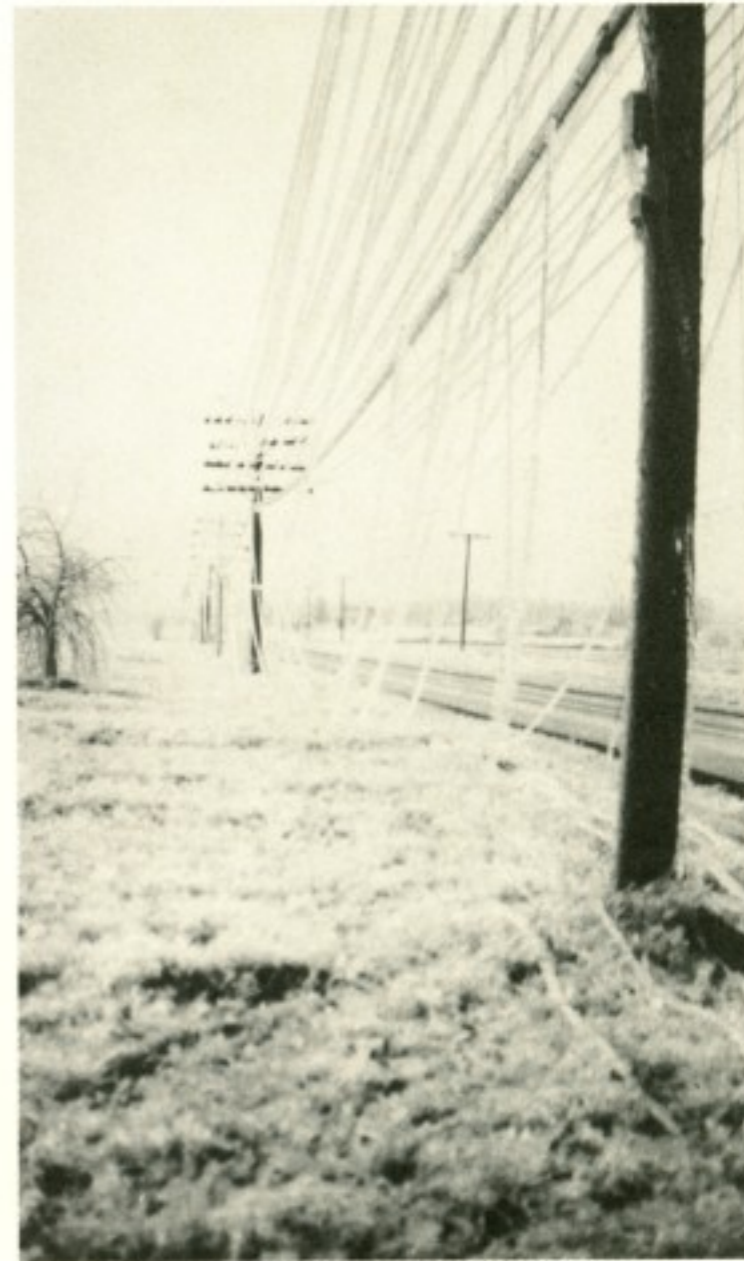
These pictures show the problems caused by ice storms during the "open wire" days.
