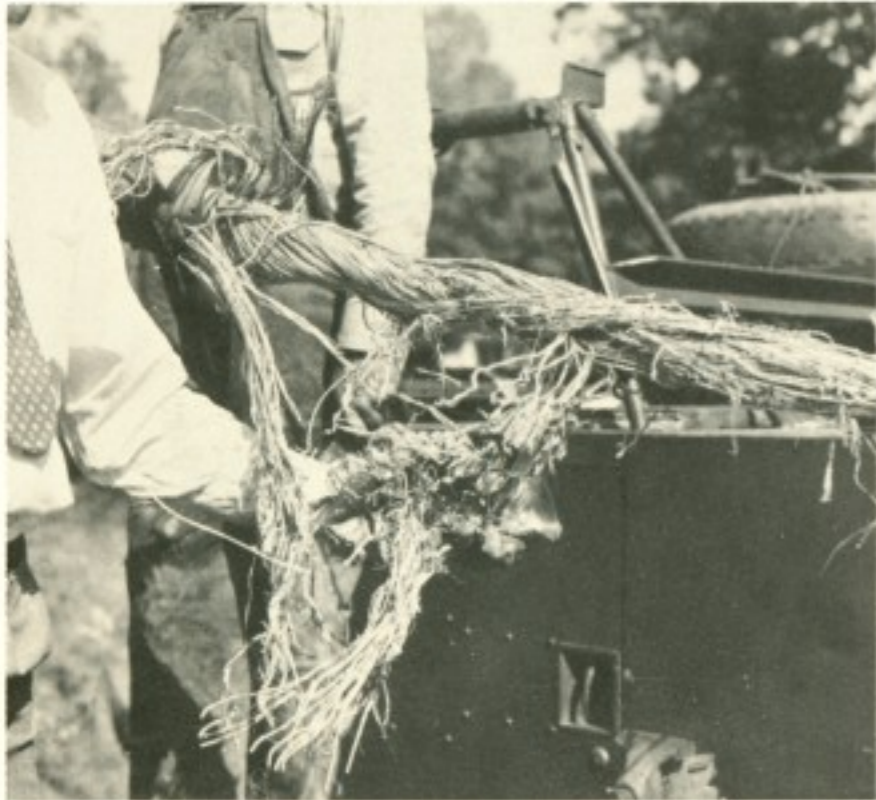
Cable damage to K carrier cable resulting from the truck which took out the pole on U. S. 1.
