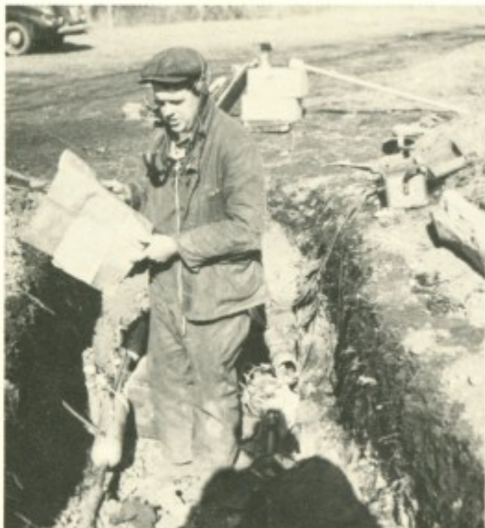
These pictures depict the installation of the Washington-Richmond "C" Cable. The job became known as "Lehman's Canal," named after the project engineer.
