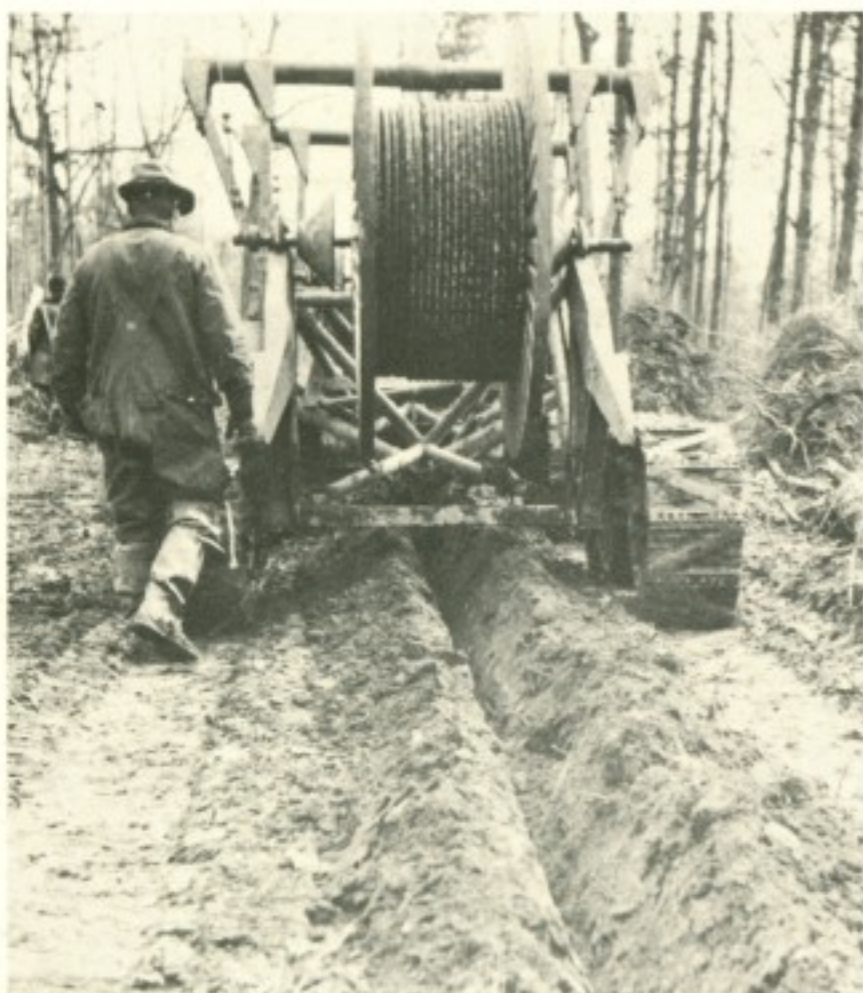
These pictures depict the installation of the Washington-Richmond "C" Cable. The job became known as "Lehman's Canal," named after the project engineer.
